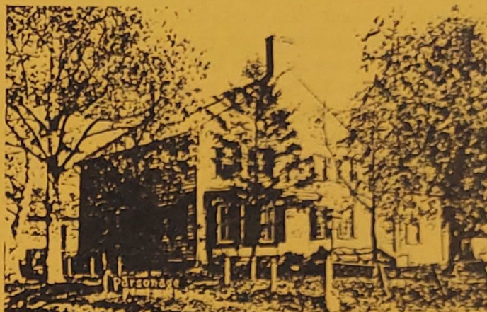
Parsonage of Penns Neck Church on Route 1. Note clapboard siding (Photo courtesy of Historical Society of Princeton.)
