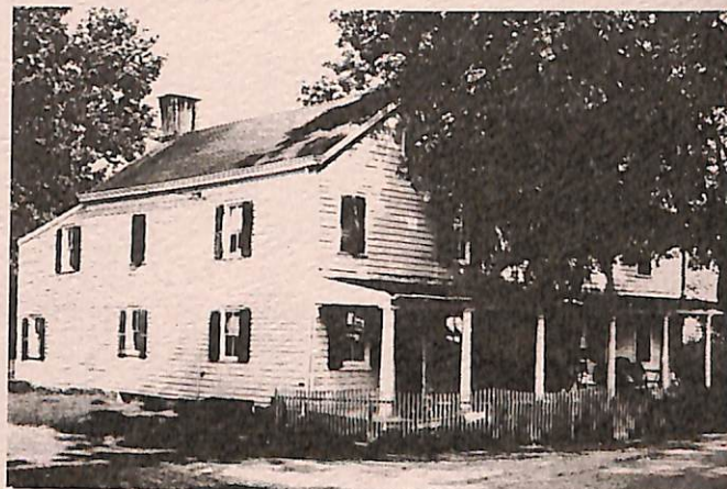
FORMER INN/HOME OF CHARLES H. MATHER, PORT MERCER GENERAL STORE OWNER. IT STILL STANDS, BUT PORCHLESS, ON QUAKER BRIDGE RD., ACROSS FROM THE BRIDGE-TENDER'S HOUSE.
