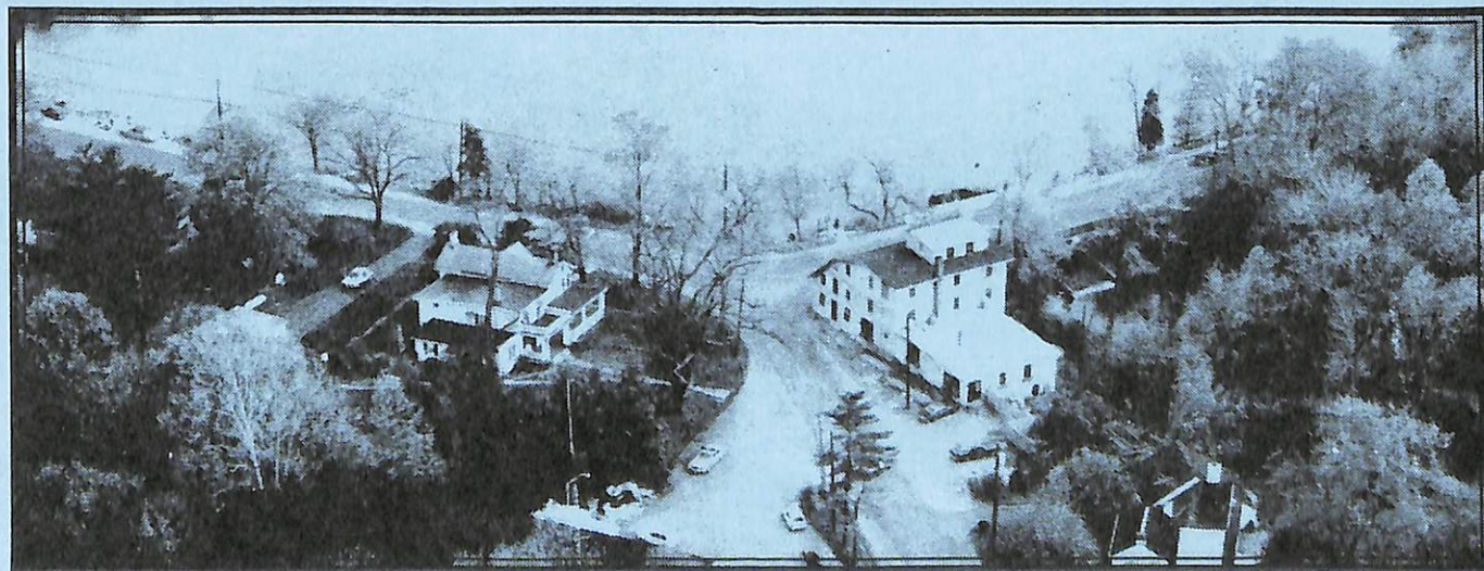
Aerial view of Grover's Mill pond & village. Mill on right; millowner's house (175 Cranbury Rd.) on left. Photo courtesy of Rossmoor News.
