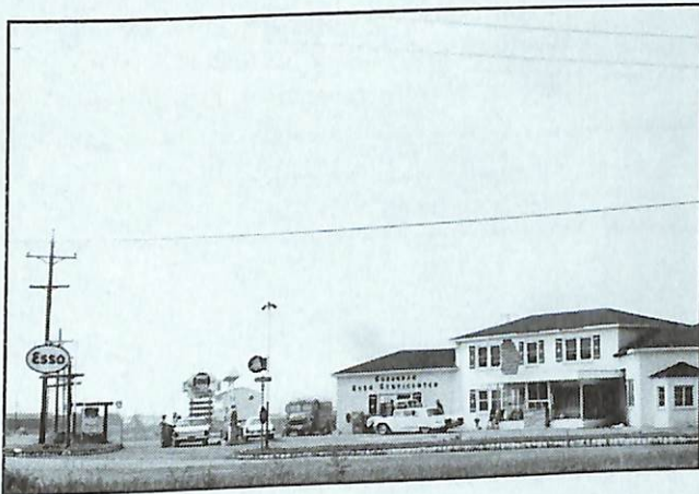
Hall's Service Station in 1962. Section at right side of the building was rented as an apartment. Service window in center of the building was used to sell frozen custard. Photo courtesy of West Windsor Township.
